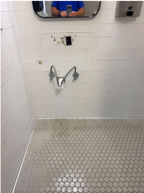
GMS removed the broken bathroom sink and cleaned the surrounding area. A new sink will be installed.
