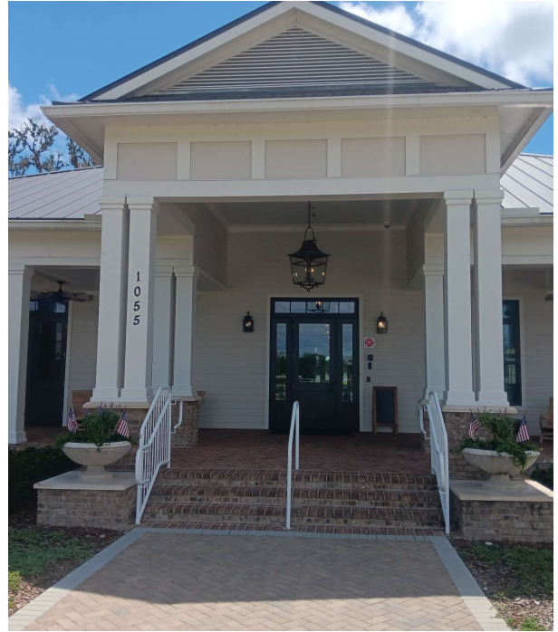
GMS pressure washed the front of the amenity building and removed cobwebs from the exterior.
